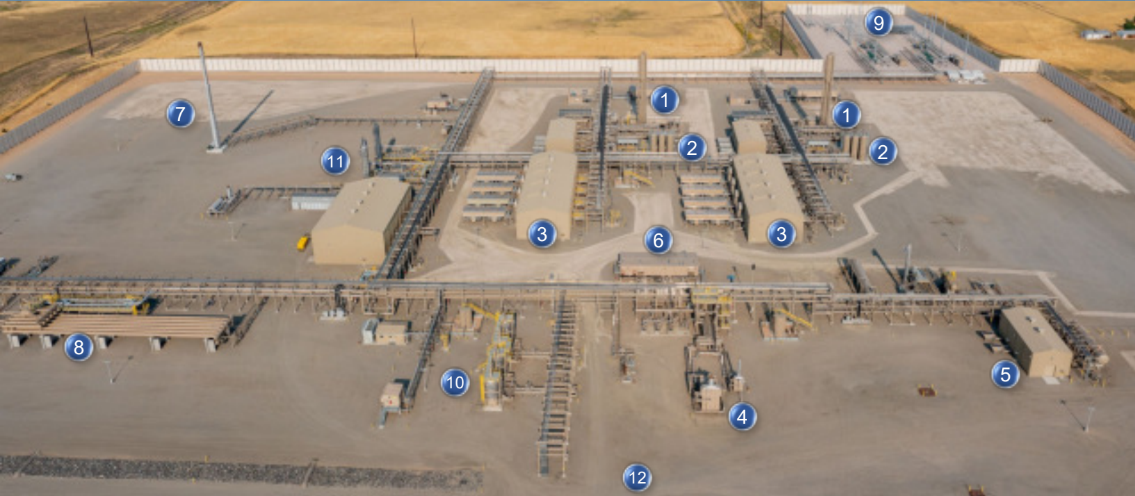
1 CRYO TRAIN Processes natural gas.
