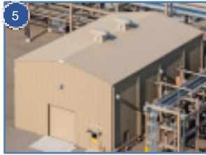
5 NGL STABILIZER Processes NGL collected in the High-Pressure Slug Catcher to meet a NGL Pipeline specification
